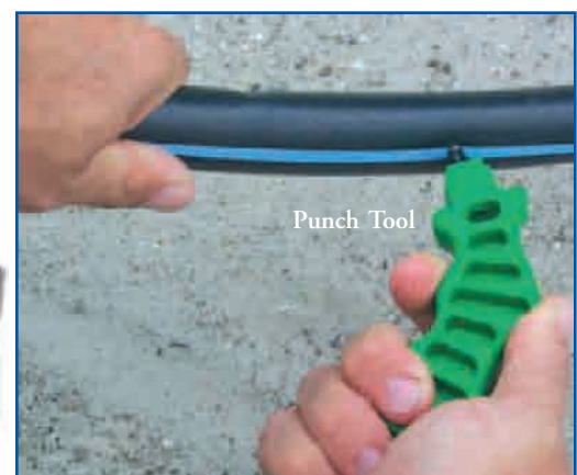
Riser Adapter Assembly
